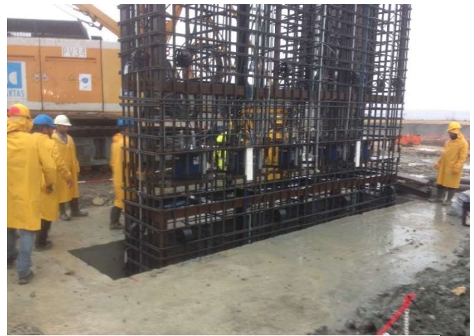
Reinforcing cage, fitted with 5 Nr 430 mm O-Cells
